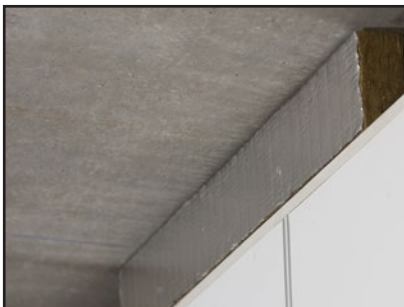
Acoustimass installed as a single 80mm thick layer
