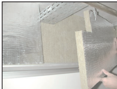
Soundstop 30 dB installed in two 30mm thick layers
